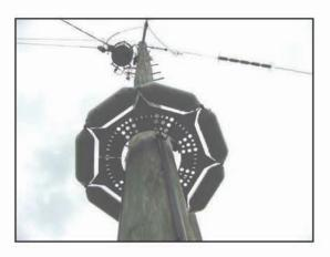
The CG POLE GUARD—Manufactured with Celcon Acetal Copolymer, one of the latest engineering resins that delivers high tensile strength and stiffness, combined with unmatched durability. This innovative design allows for a high level of lubricity over a broad range of temperature, and chemical environments. This exceptional system of dimensional stability, merged into a hard, high gloss finish, will always deliver the solution that saves.
